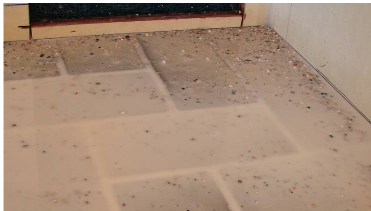
c) Adding water to soak fine material into the joints
