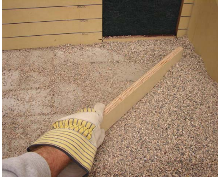
Figure 8: Applying joint material
