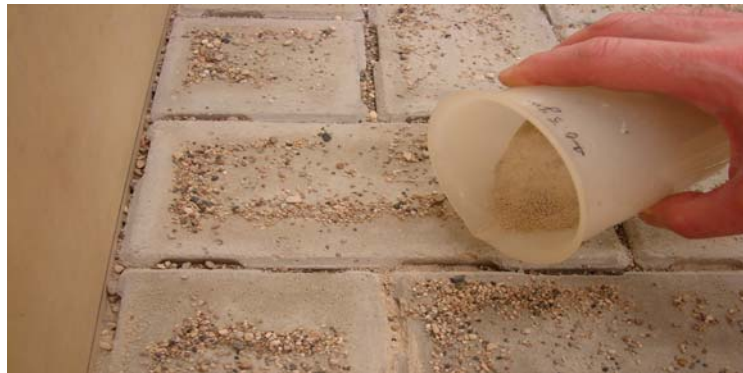
b) Placing fine material (passing 850 \mu\text{m} (No. 20) sieve size)
