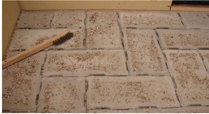
a) Brushing out top 4 to 6 mm of joint sand
