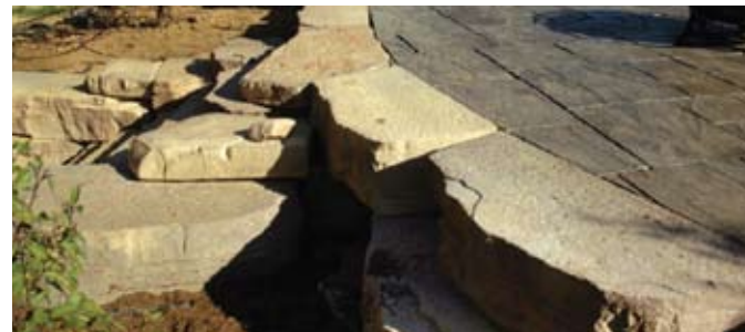
Place pavers flush with the back of the Rosetta Blocks
