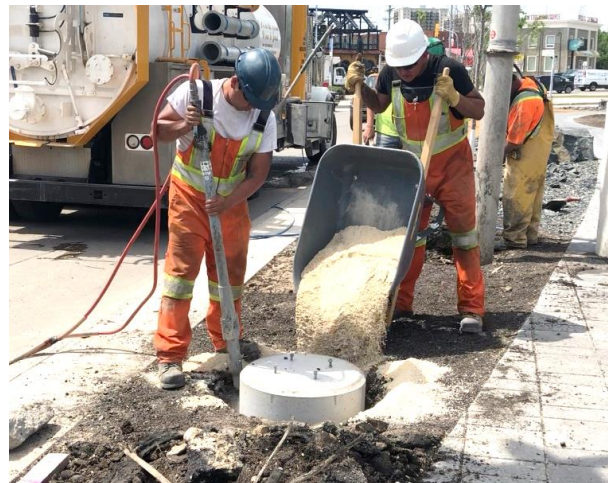
Photo 4: Place backfill and compact with pole tamper.
