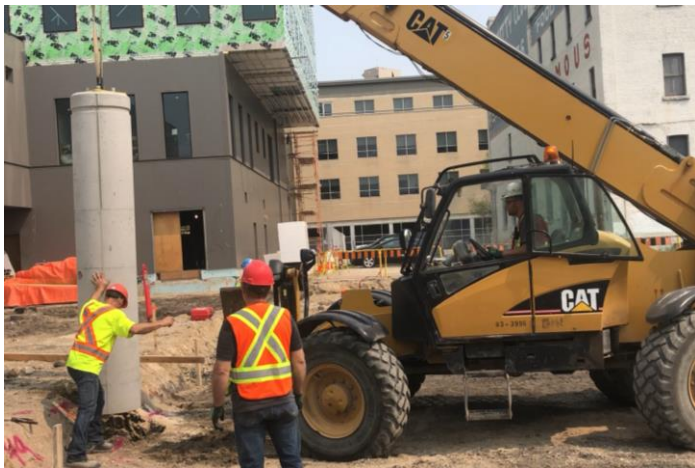
Photo 3: Lower Unit into hole
