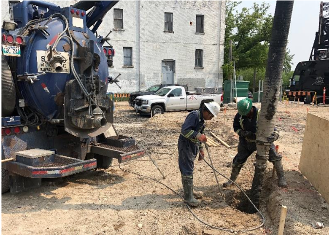
Photo 1: Auger or HydroVac Hole.
